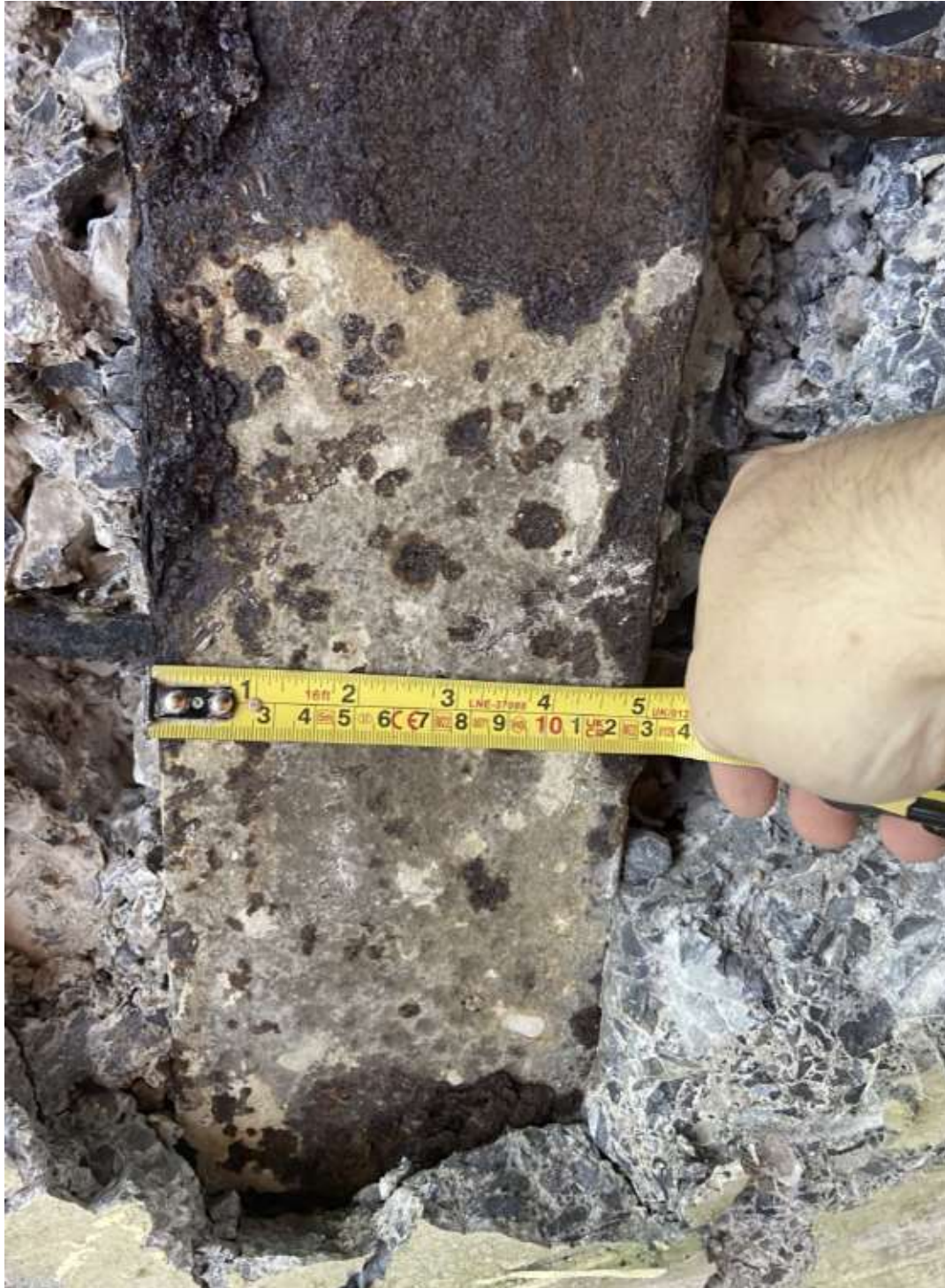
Figure 42: 125mm wide bottom flange of internal beam
