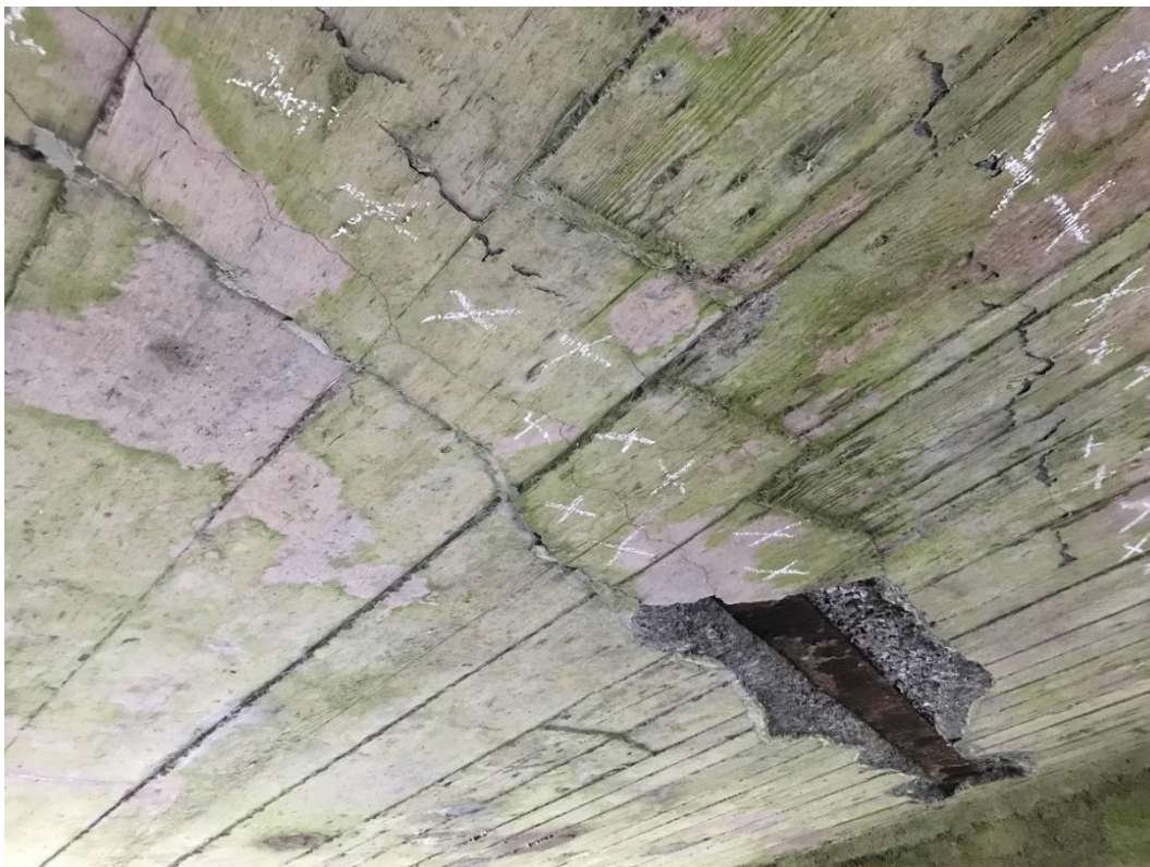
Figure 3-2 - North span with spalling, delamination and exposed filler beams evident
