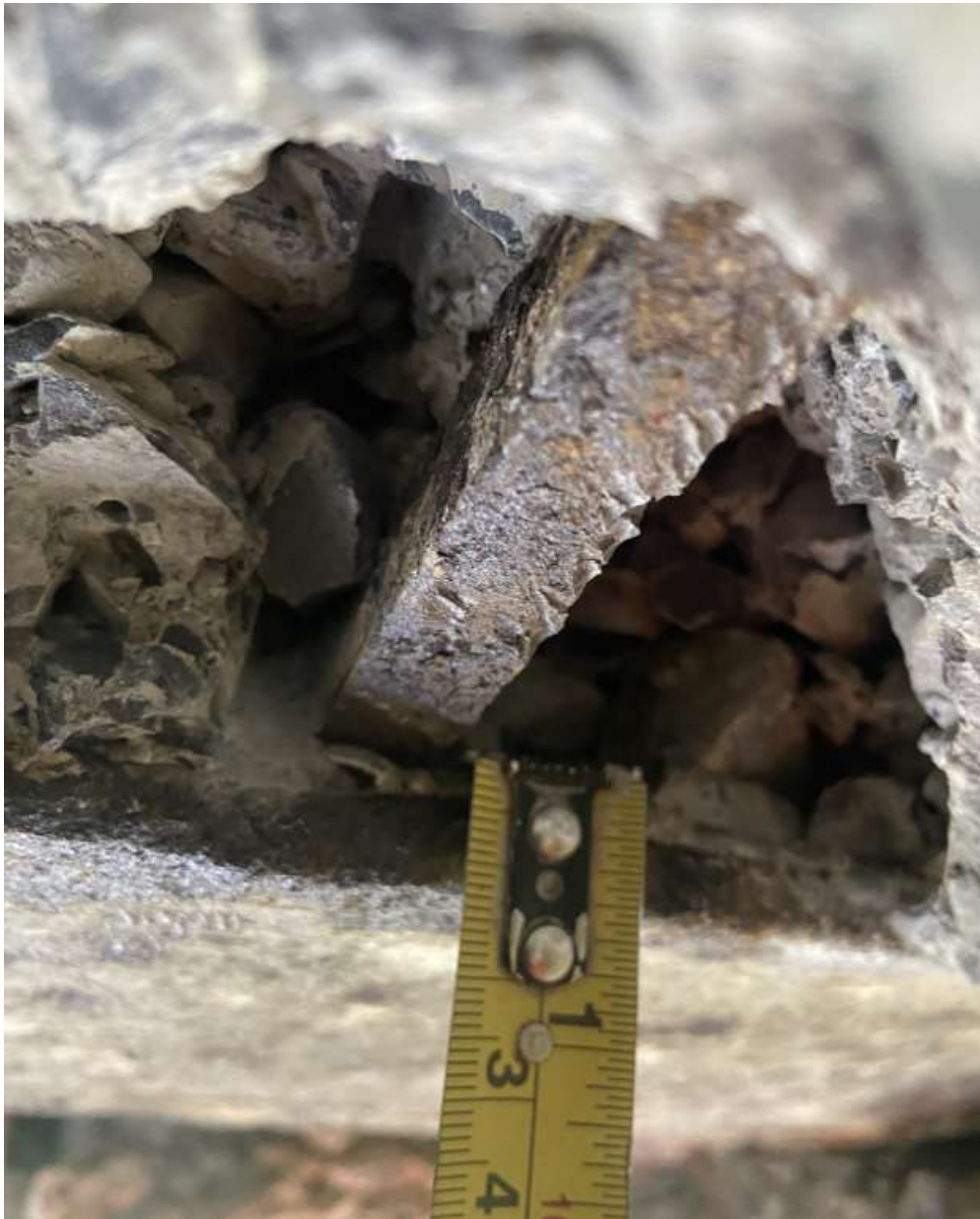
Figure 40: Longitudinal bottom flange thickness
