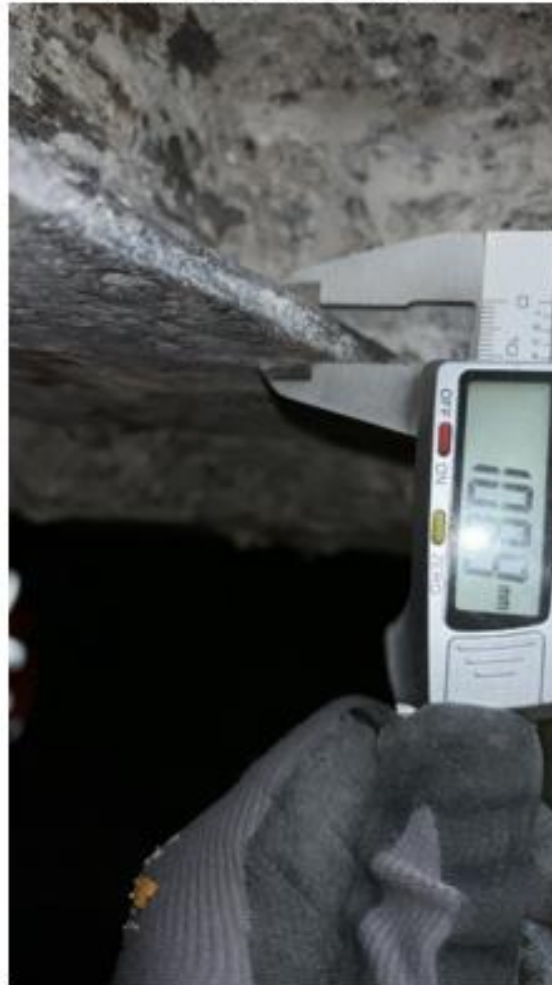
Area 3 - Bottom flange 124mm width
