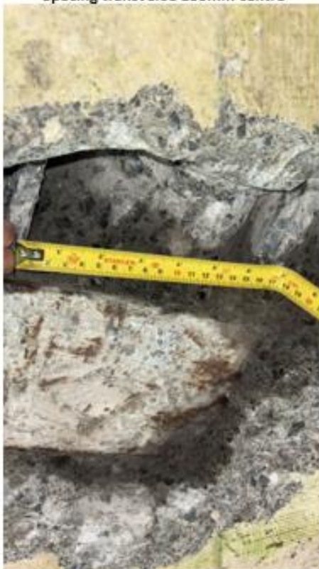
Spacing transverse 160mm centre
