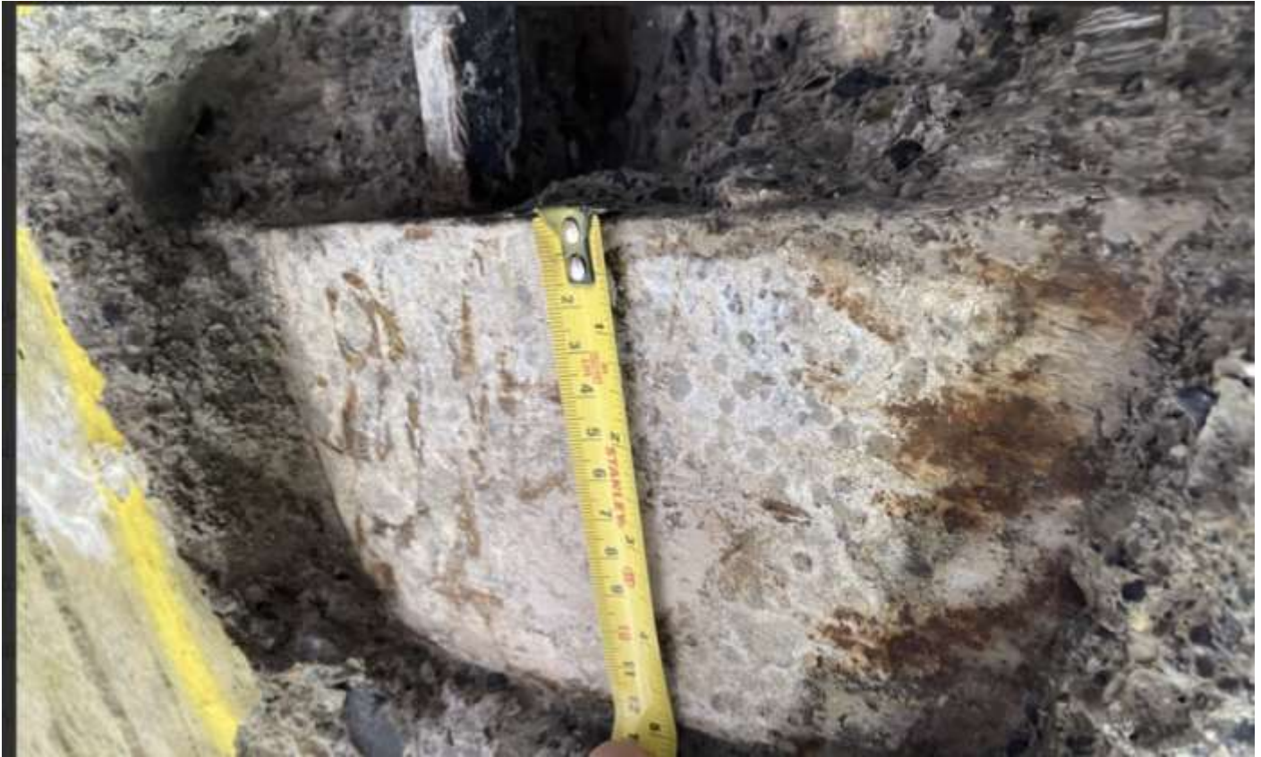
Figure 25: Measurement of longitudinal beam flange
