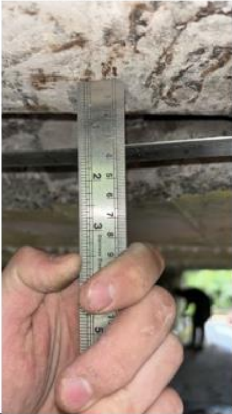
Cover bottom flange 34mm
