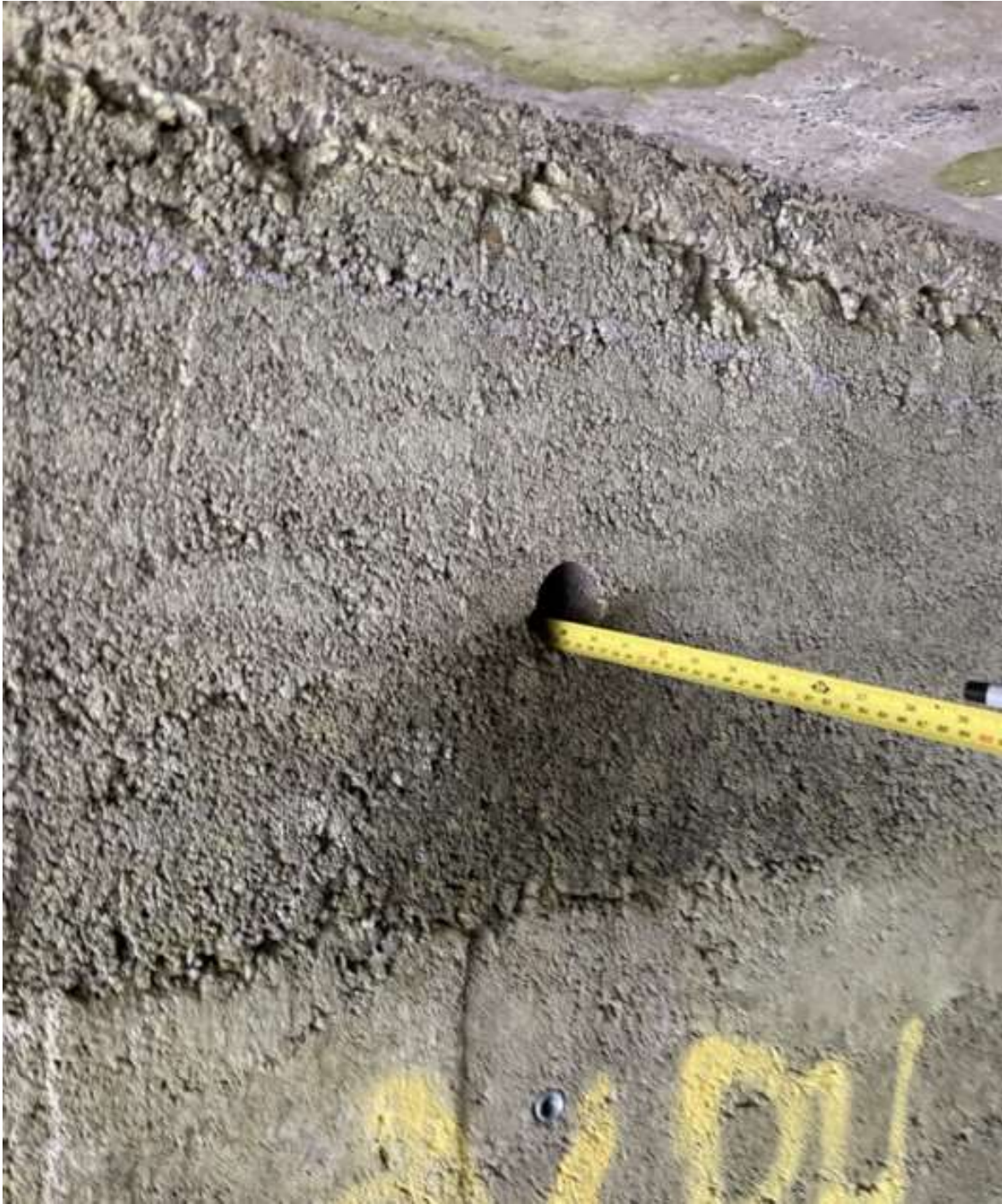
Figure 45: Pilot hole depth measurement
