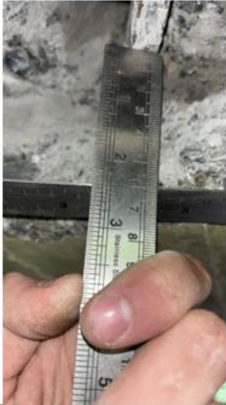
Cover transverse square rebar 59mm
