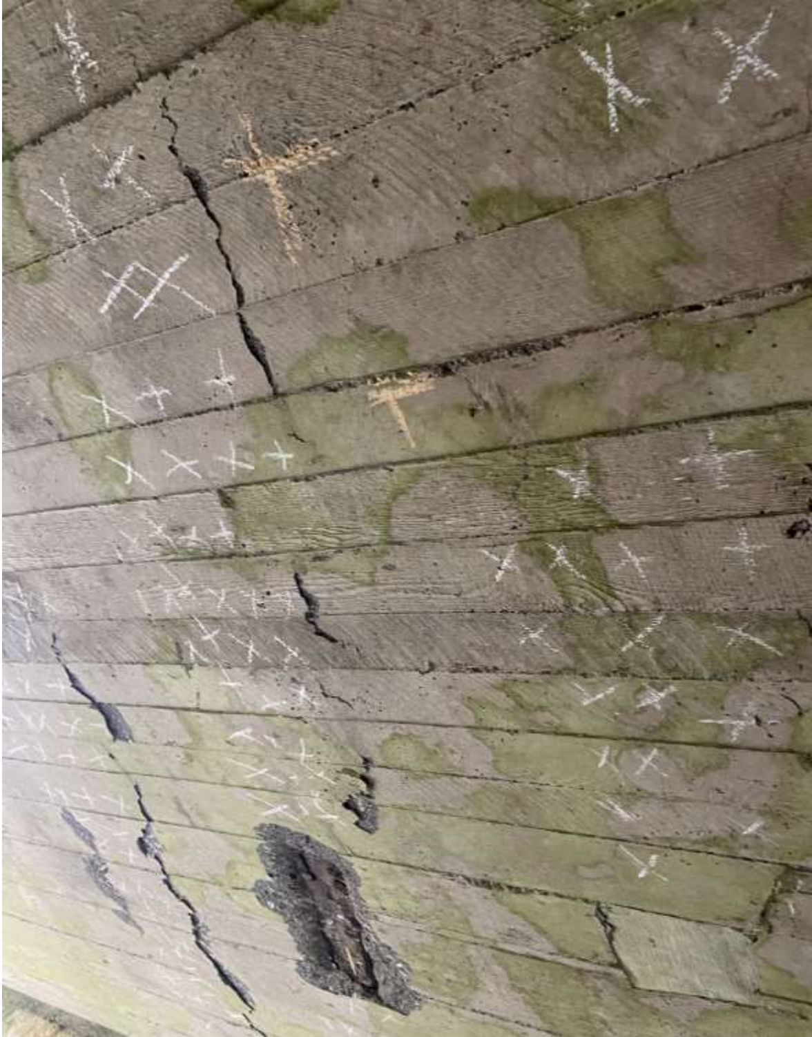
Figure 29: Further delamination on south arch
