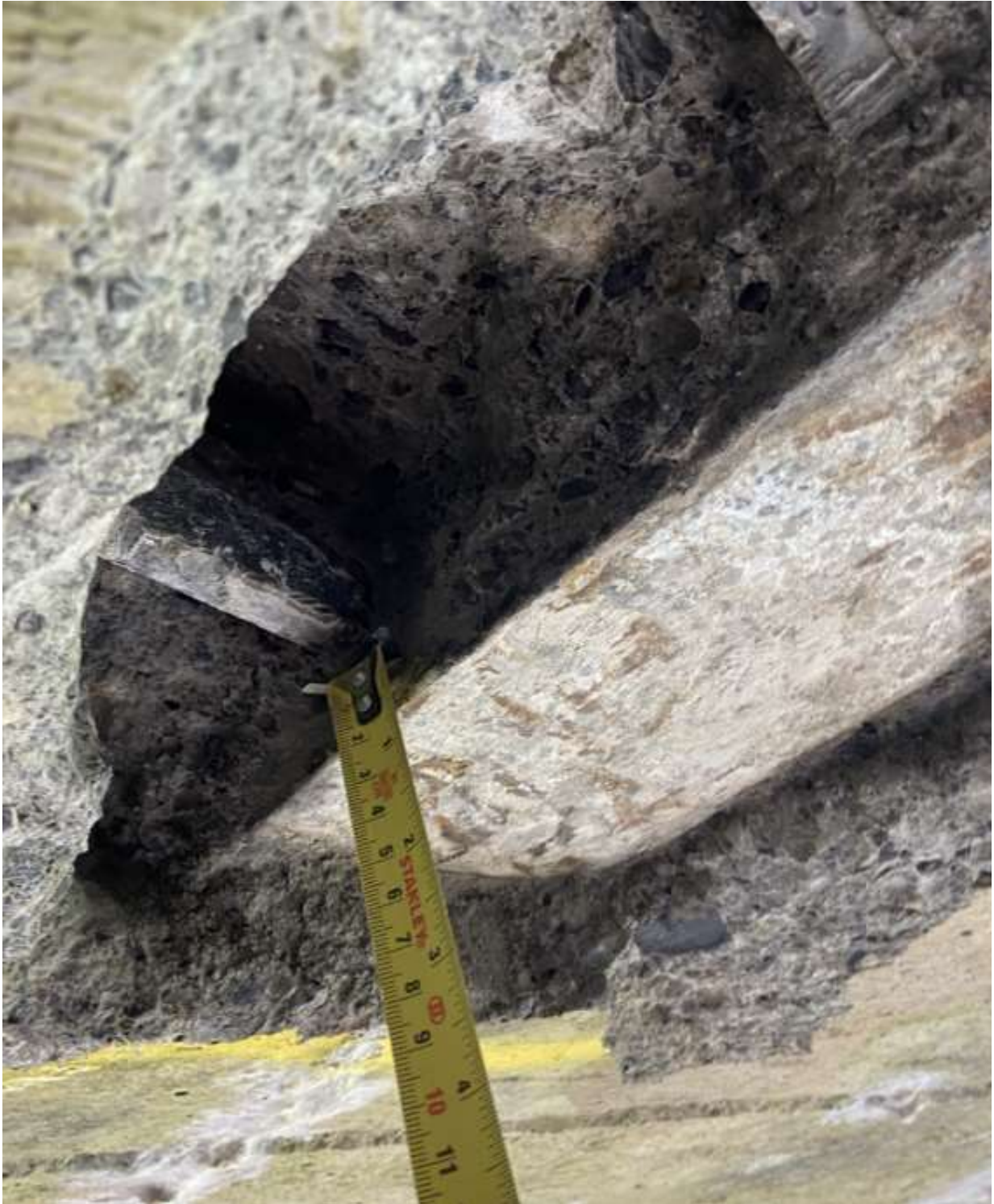
Figure 26: Transverse steel members running perpendicular to longitudinal members at 160mm spacing
