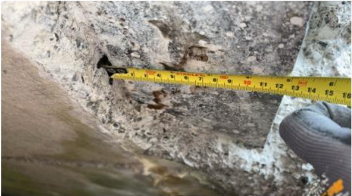
Area 3 - Bottom flange 124mm width
