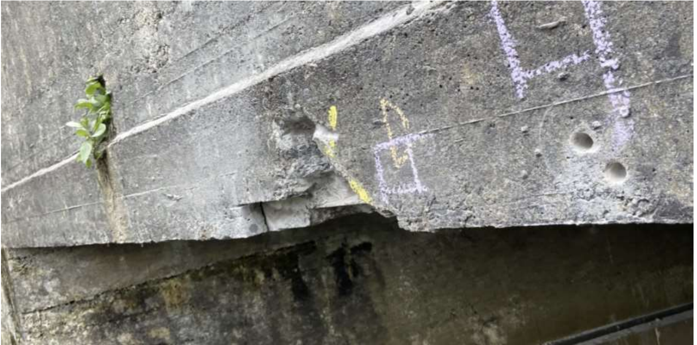
Figure 34: Breakout at test area 4 exposing external beam
