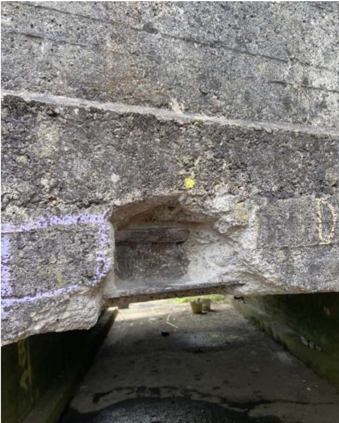
Figure 20: Breakout of external beam
