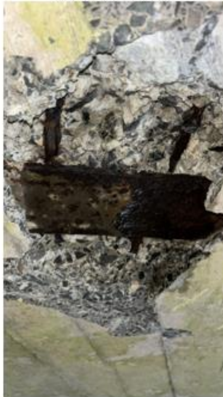
Area 4.1 soffit breakout
