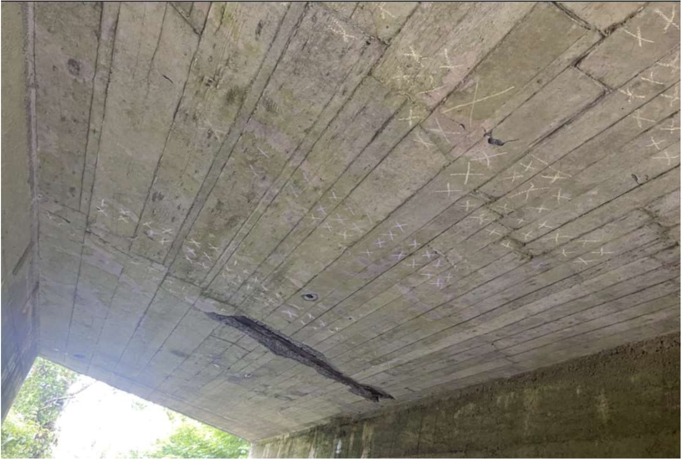
Figure 38: Delamination survey in Northern arch wide angle view
