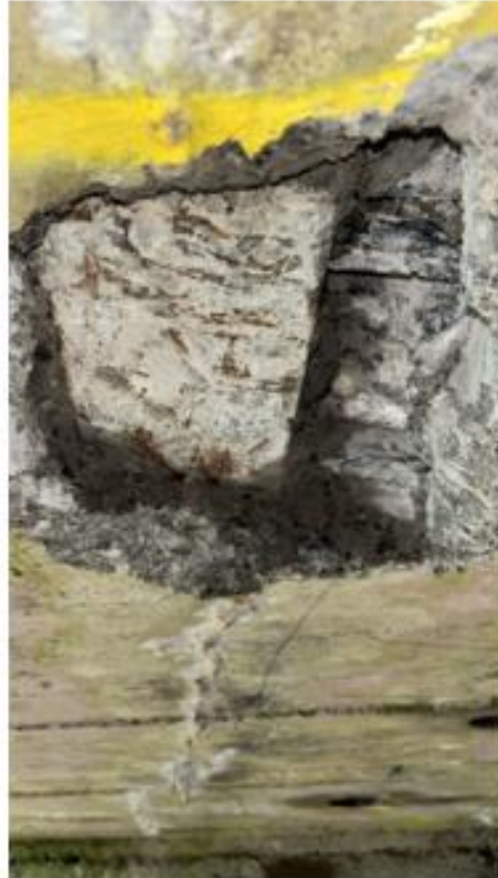
Area 3.1 Soffit breakout
