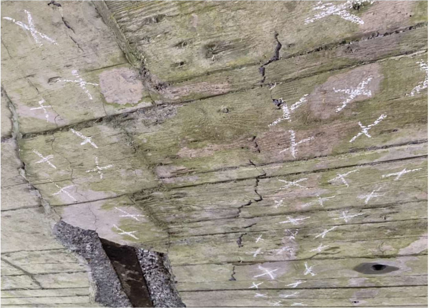
Figure 37: Delamination found in northern arch
