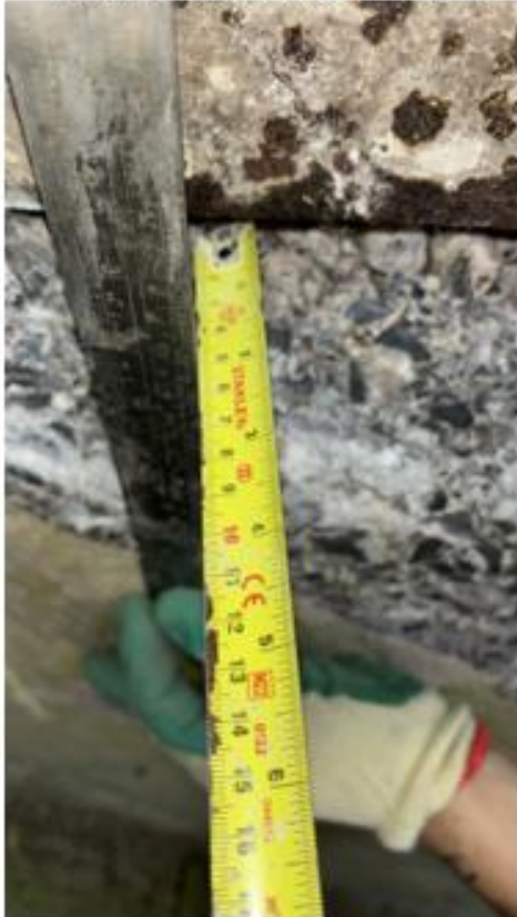
Transverse square rebar cover 51mm
