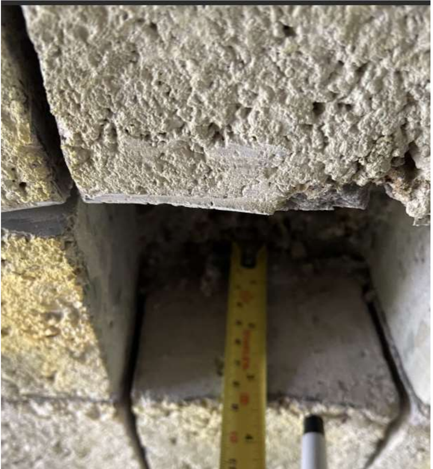
Figure 49: TA6 carbonation sample depth into pier
