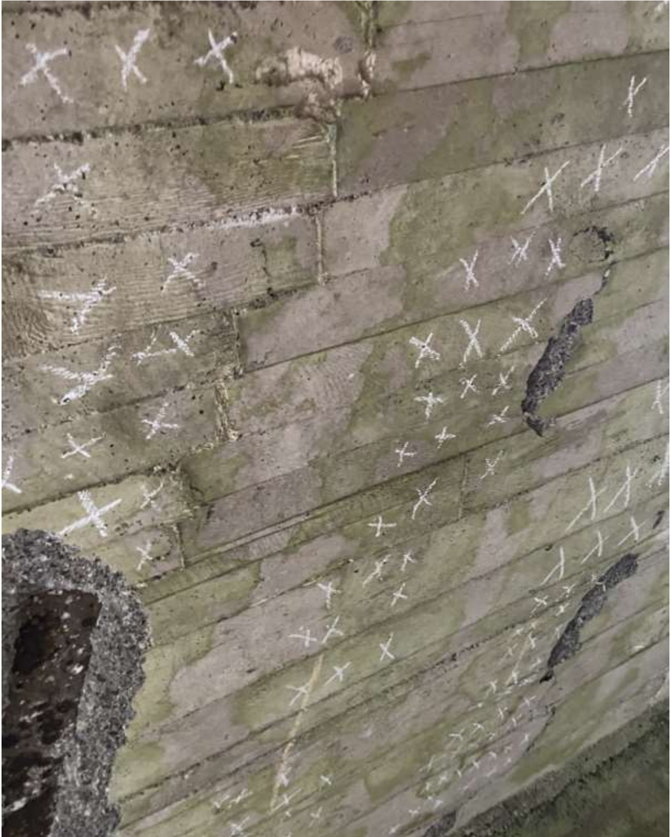
Figure 30: Exposed beams due to delamination of concrete cover
