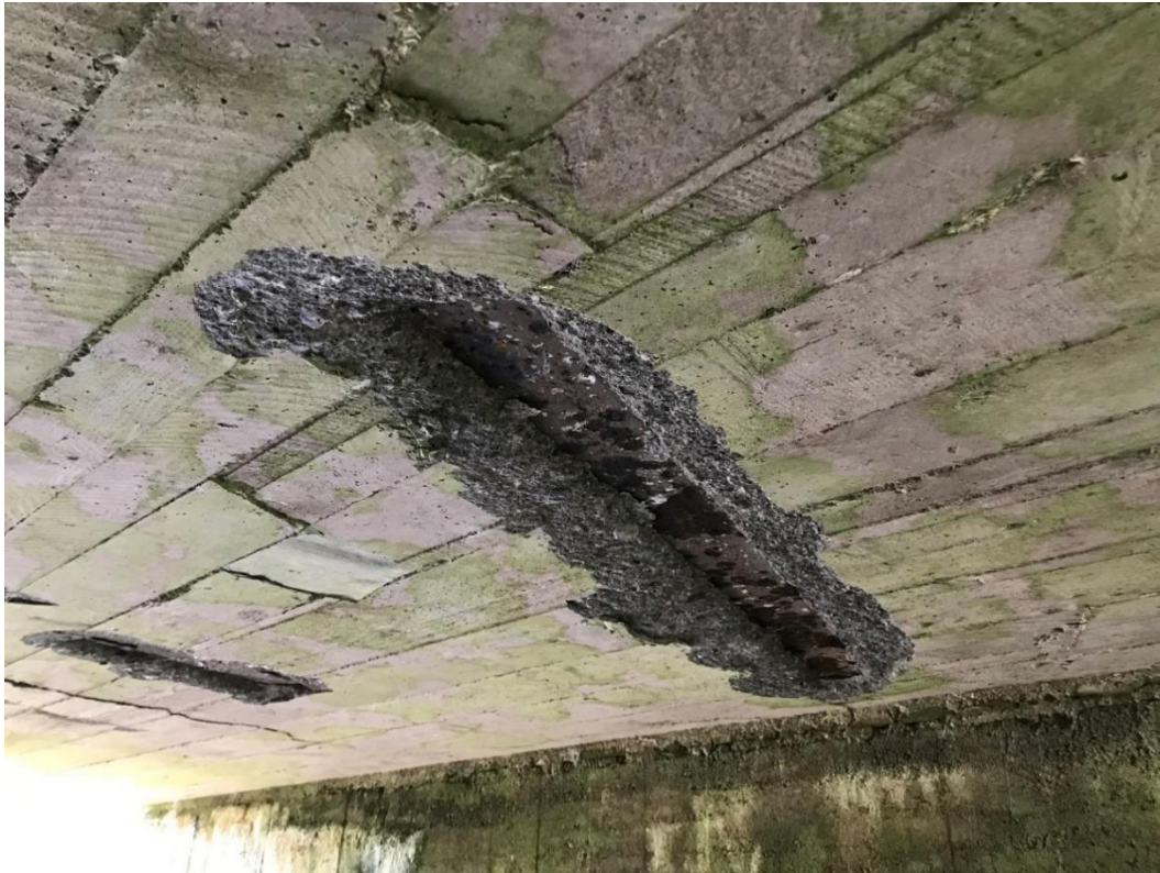
Figure 3-1 - South span with spalling and exposed filler beams evident
