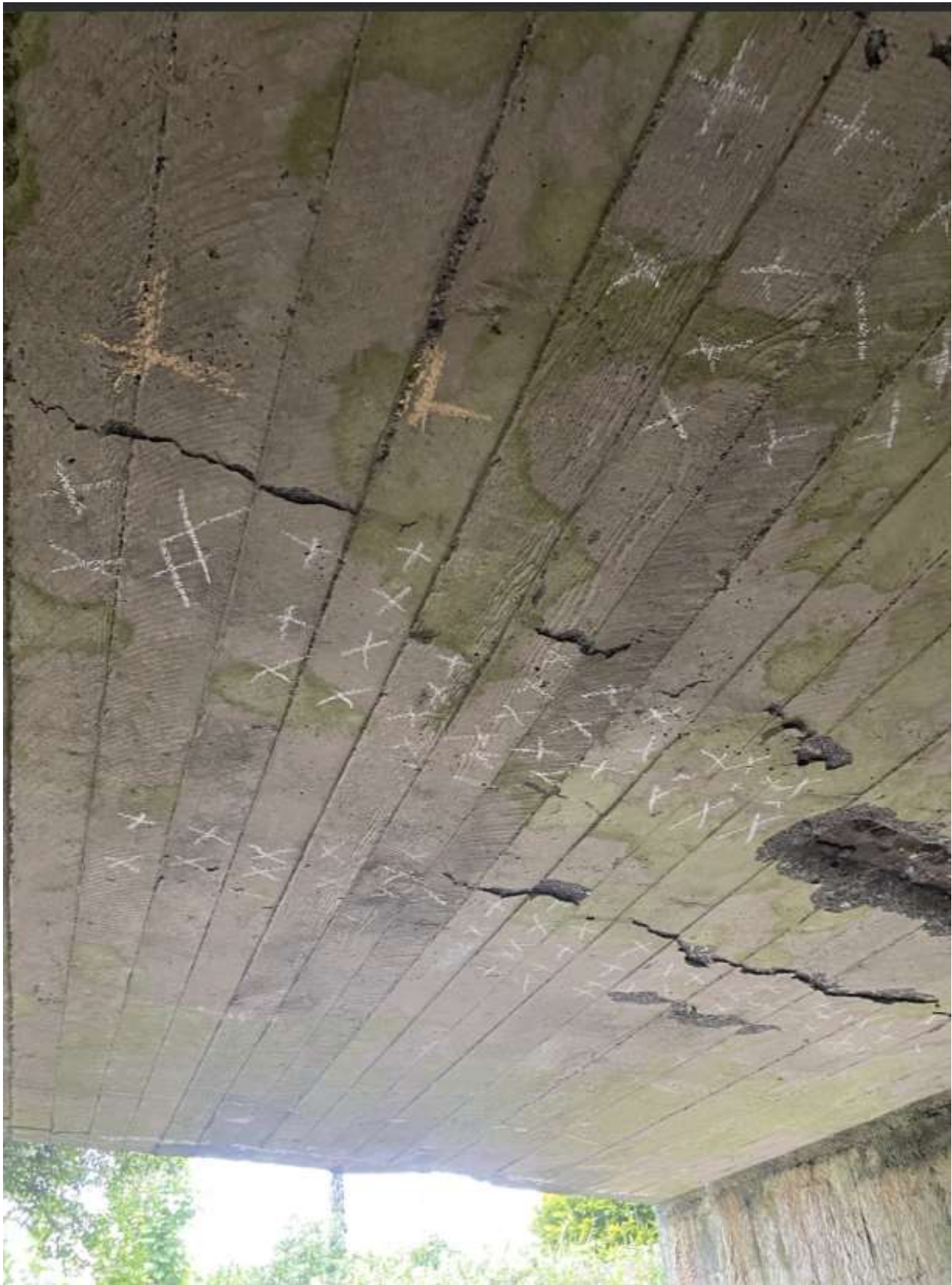
Figure 28: Delamination survey showed significant delamination underneath longitudinal sections on south arch
